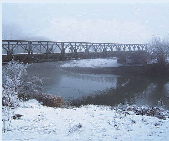
The bailey bridge built to replace the old drawbridge to the Ings
