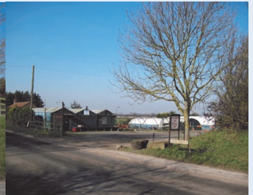
Disused nursery buildings.
